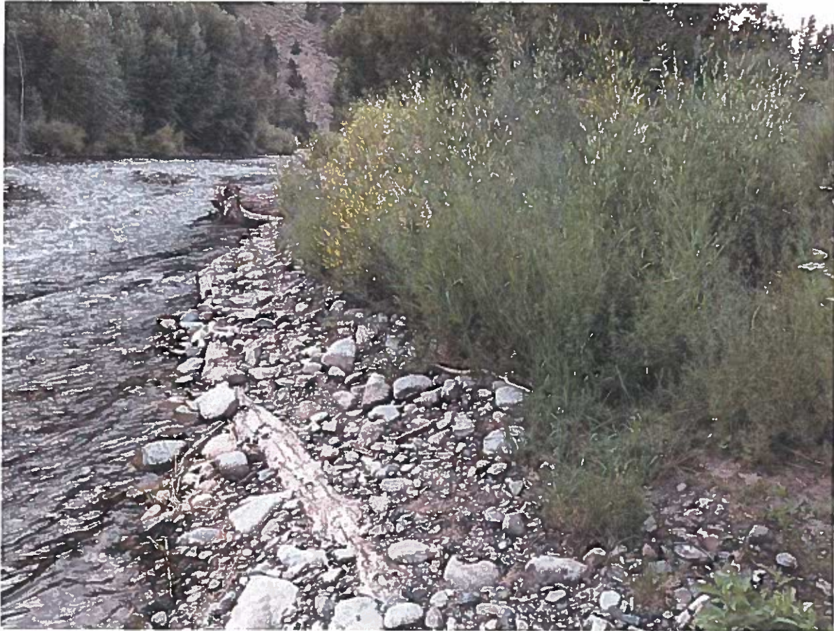
Photo 1: Similar to Proposed Streambank Reconstruction and Stabilization on Big Wood River
